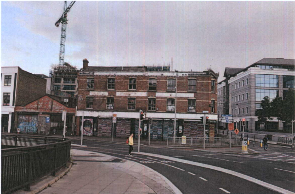
Plate 1. Proposed development site (main building)
